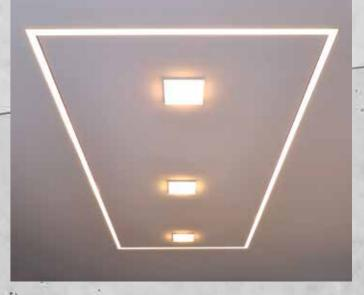
After casting the concrete and removal of the formwork panels with the multiplex boards, the shape of the light line becomes visible. Now the linear individual luminaires can be inserted into the concrete installation profile PALERMO BE. The magnetic holders ensure that the corresponding luminaires fit precisely and securely in the right place.
