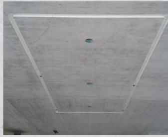
Align the supplied multiplex boards exactly to the desired light integration points and screw them tightly to the formwork. Then press the concrete installation profile PALERMO BE onto the multiplex board and fasten it with the screws supplied..
